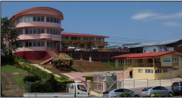
The new Diocesan building sits alongside St John the Baptist Theological College and the new carpark has been built in front of the original college building
